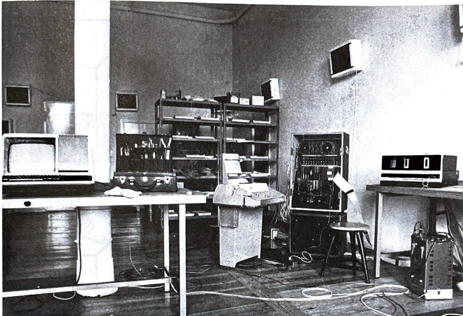
Figure 11.2 Edward Kobrin's HYBRID IV studio set up in Berlin, 1977, featuring a computer-controlled 16-channel spatialization system. The loudspeakers are mounted on the walls.
