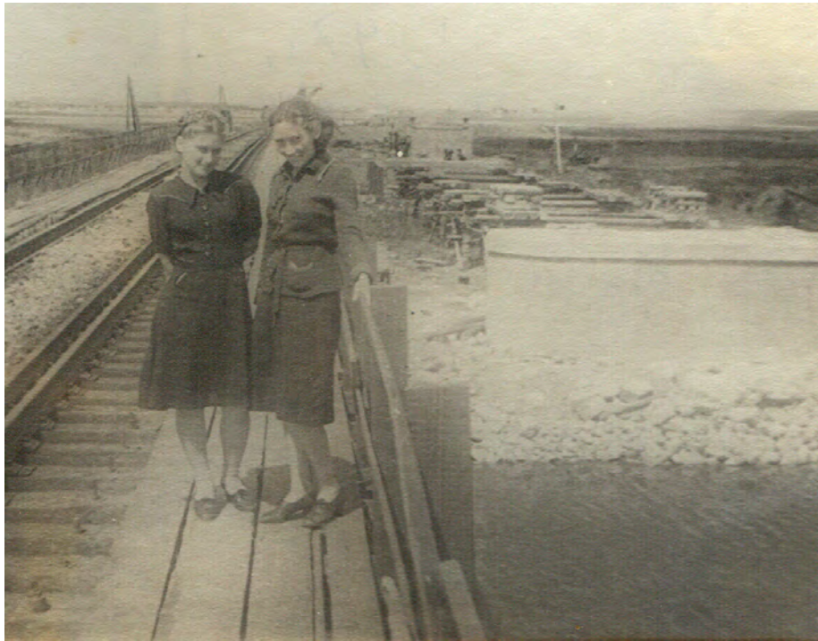
(6). Anya (left) and Nadya on the bridge they constructed.
